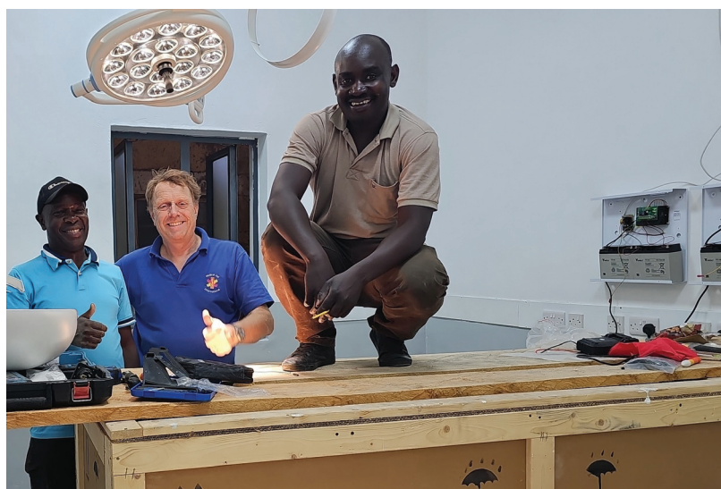
Tim Beacon working with MedAid trained biomedical engineers in Kenya, installing and commissioning an operating room.
